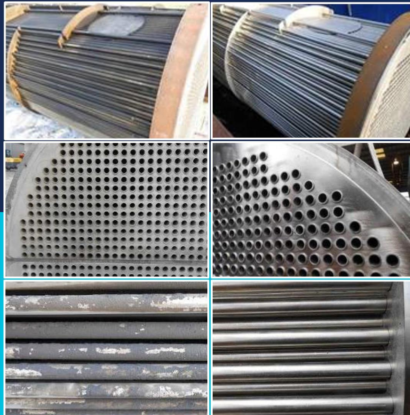
FIGURE 4. BEFORE AND AFTER PHOTOS OF ONE OF THE EXCHANGERS CLEANED
